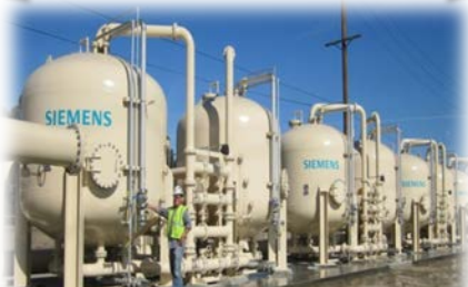
SF Groundwater Basin Remediation
