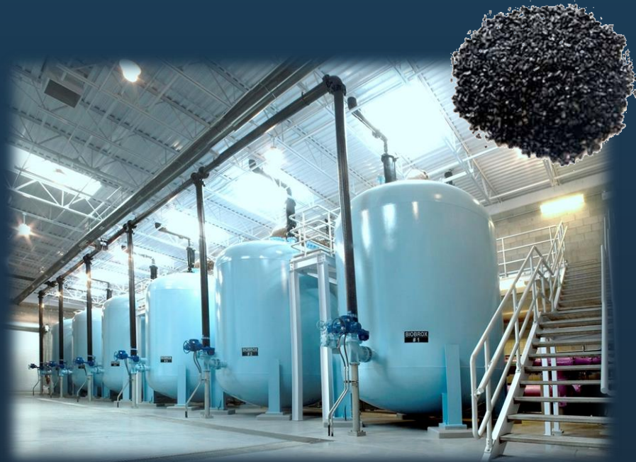
Carbon Adsorption: Granular Activated Carbon (GAC)
