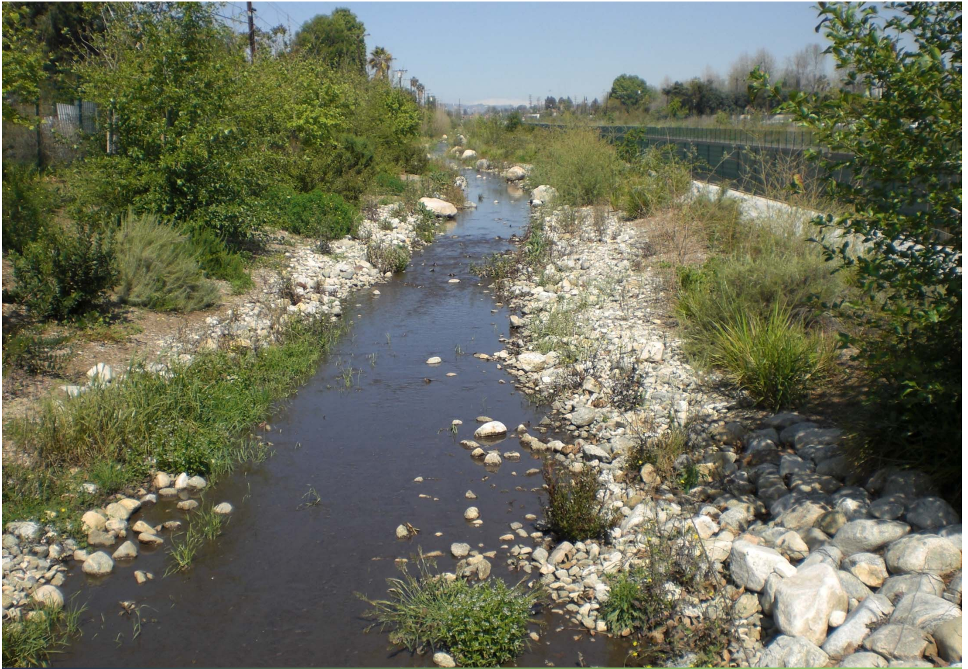
Tujunga Wash Greenway and Streambed Restoration
